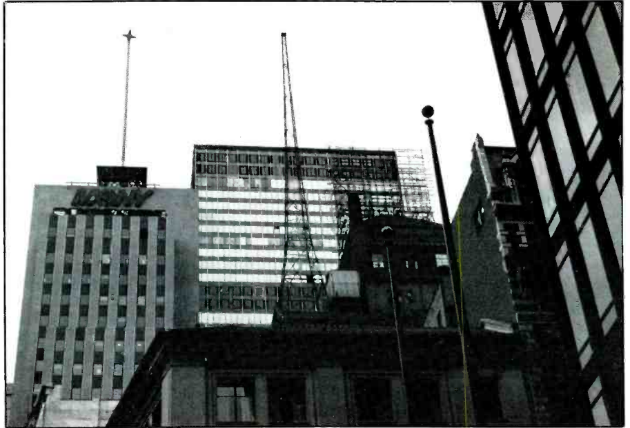
The radio tower in the middle of this photo was used by old time station WPCH, which existed in New York City in the 1920's. The tower hasn't been used for more than sixty years, and is probably the last existing AM broadcast tower in Manhattan. (Courtesy Chris Edwards, N.J.)
